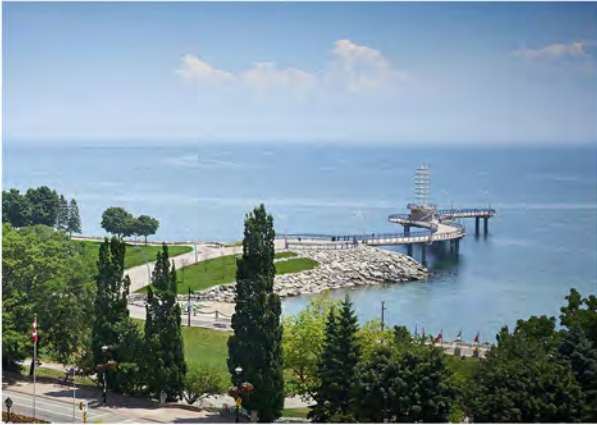
PIER IN BURLINGTON, ON
